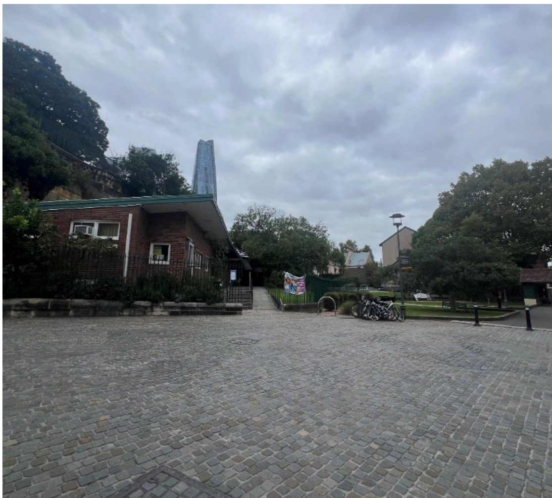
Site viewed from Watson Road
