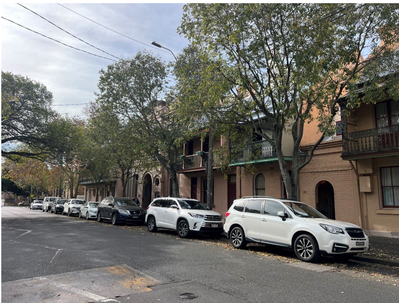
View of terrace housing on Kent Street (rear boundary to subject site, viewed from western side of Kent Street
